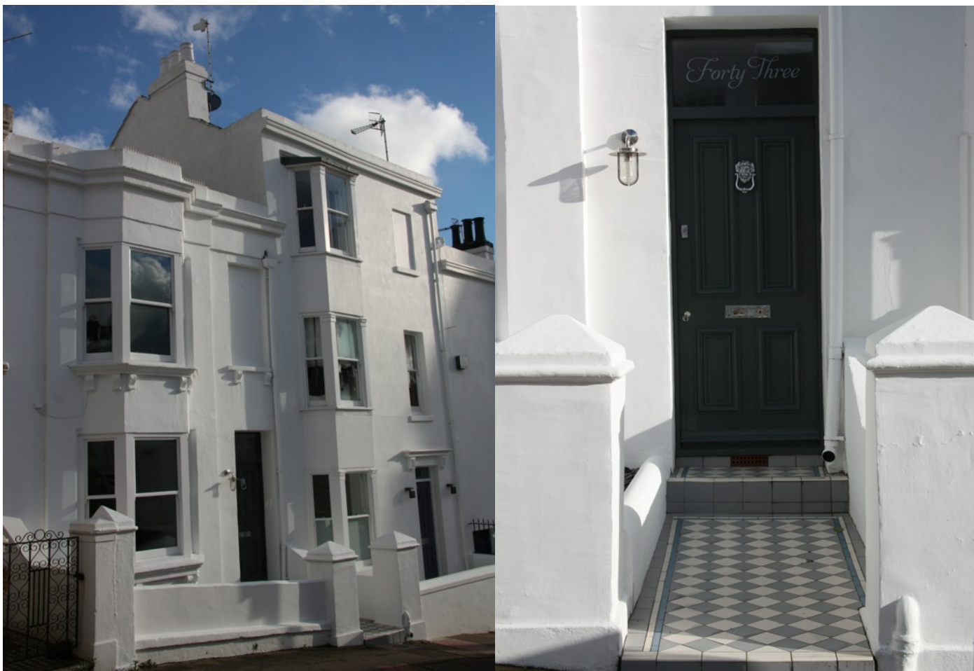
Next door neighbours: 43 and 44 Victoria Street with a close-up of the path at 43 (right)
