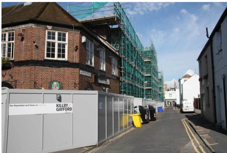
Ghostly site: work has stopped on the conversion of Mitre House
