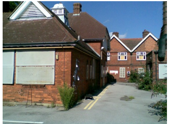
Take a last look: all these buildings will go
