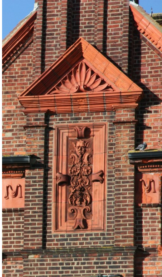
Terracotta detail on the south facade
