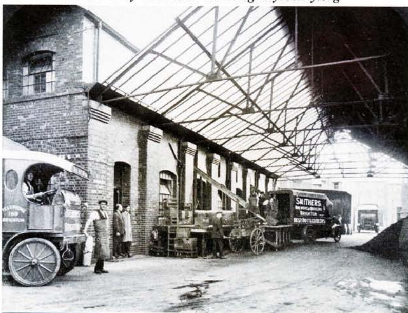
OFFICE AND LOADING DOCK. BOTTLING STORE.
